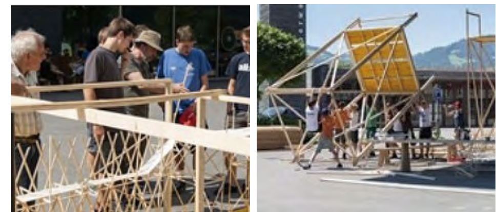
Werkraum School students building a structure of wood, supported by design teachers, coaches and craftsmen. Learning Lab 2019. © Roswitha Schneider
